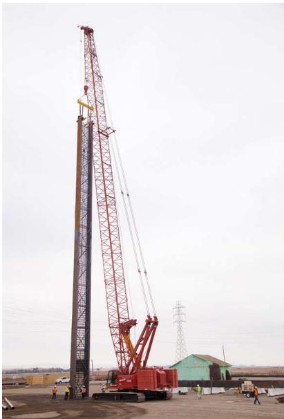
Lifting steel cage for the shaft wall.
