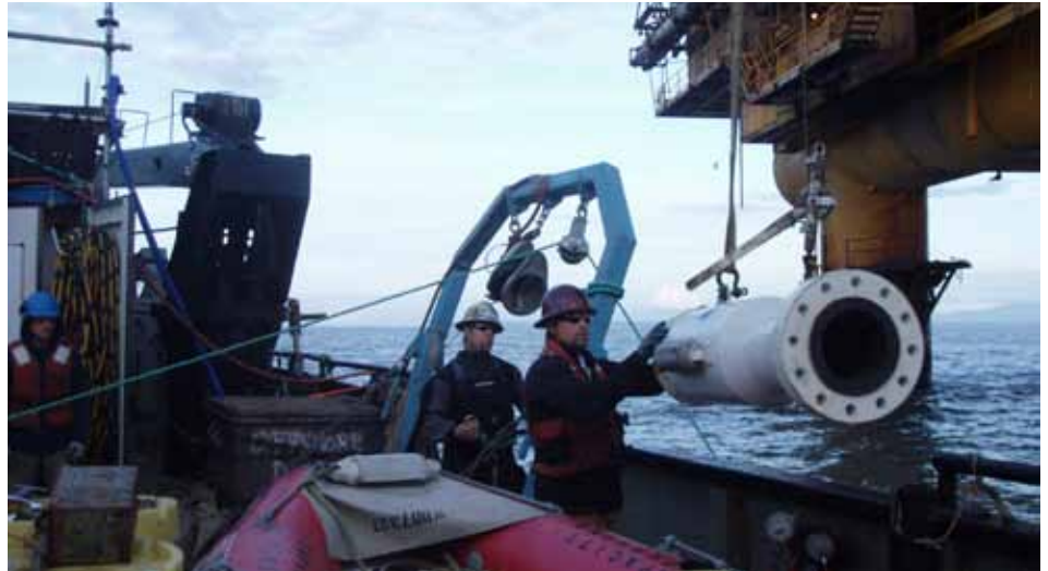
Jake Elhard and Josh Pool prepare spool piece for installation
