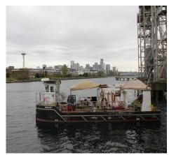
Global was contracted to install protective wrap and steel jackets to the intertidal area of the steel pilings that support Grain Terminal 86 on the Seattle waterfront.
